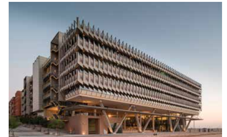
The Siemens Headquarters is the first building in Abu Dhabi to achieve a Leed platinum rating. © Masdar.
