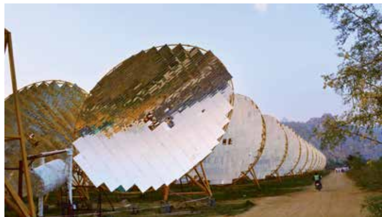
India One Solar Thermal Power Plant, Aburoad, Rajasthan, India.
