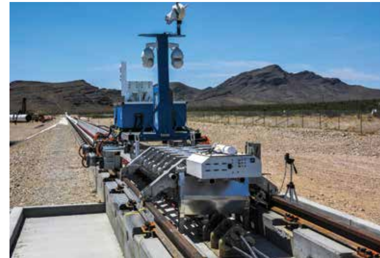
The first test of the propulsion system at the Hyperloop One Test and Safety site in May, 2016 in Las Vegas. © Hyperloop One / Bjarke Engels Group.
