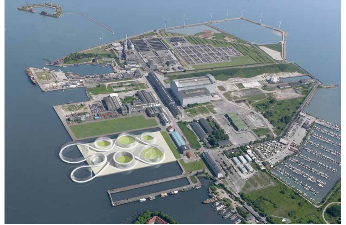
eMotions creates ten different outdoor rooms, each highlighting a unique mix of renewable energy generating technologies.
