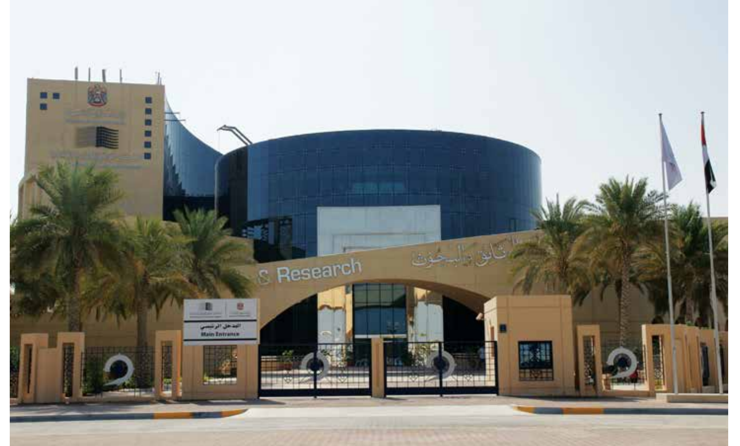
The National Archives of the UAE building in Abu Dhabi. © National Archives.
